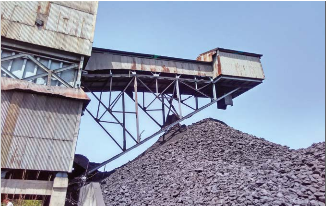
Site Photo : Structural Adequacy Study for Bina CHP, NCL.
