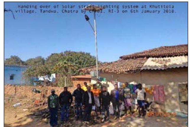
Fig: Installed solar lights in Chatra, Jharkhand
